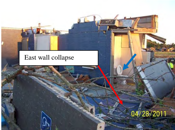
Figure 5 (Figure 7-53 of the MAT Report): View of the collapsed east wall (red arrow) and restroom (blue arrow) of the Smithville Police Department. Note that some of the restroom walls collapsed (Smithville, MS)
