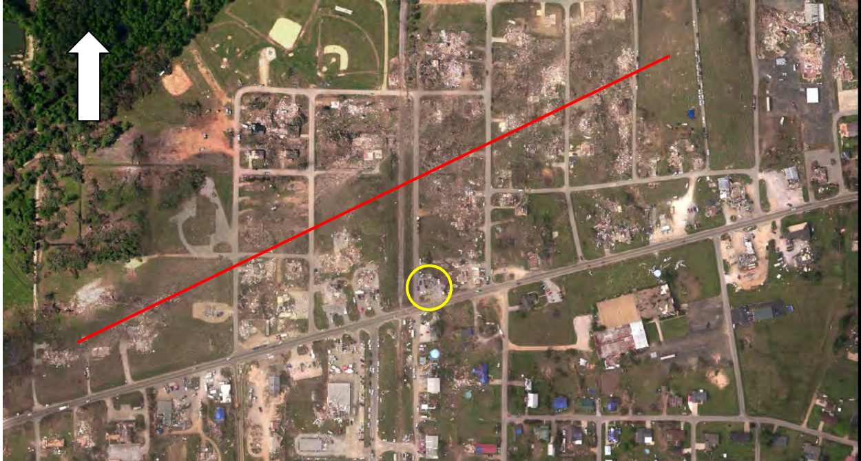
Figure 3 (Figure 7-48 of the MAT Report): Aerial view of the tornado track in the vicinity of the Smithville Police Department (yellow circle). The center of the track is approximated by the red line (Smithville, MS) (Source: Modified from NOAA, 2011)
