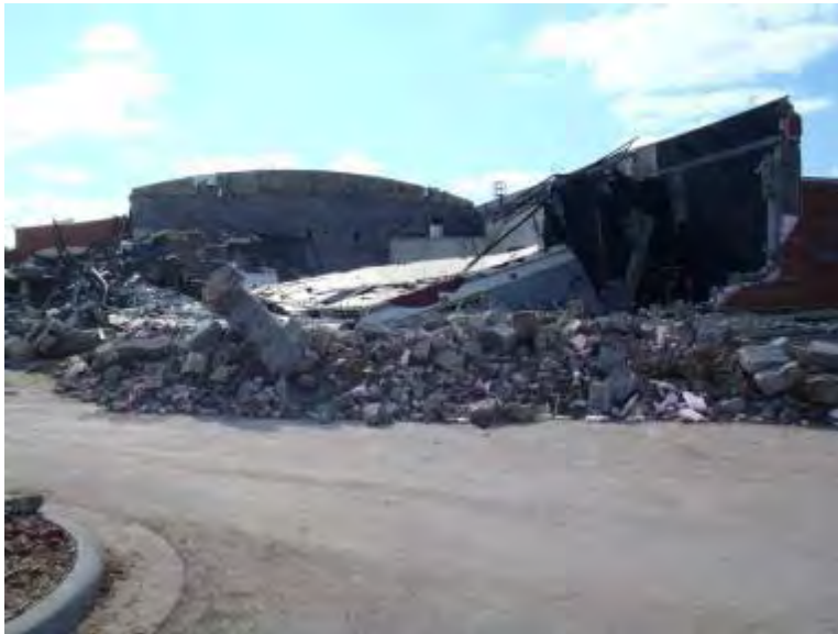
Figure 1 (Figure 6-44 of the MAT Report): View of the collapse of the auditorium roof and both exterior walls of Joplin East Middle School.
