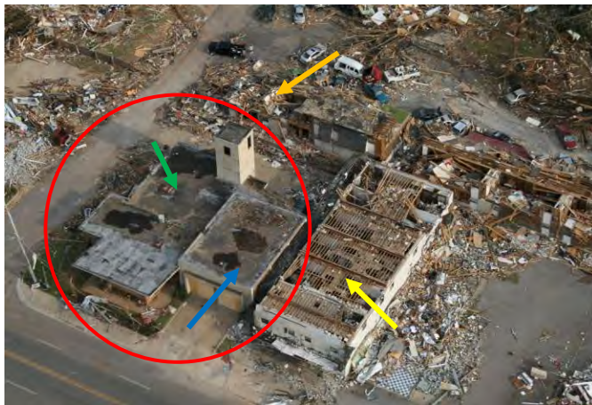
Figure 2 (Figure 7-39 of the MAT Report): The fire station is within the red circle. The apparatus bay is indicated by the blue arrow and the living quarters are indicated by the green arrow. The yellow and orange arrows indicate the nearby heavily damaged apartment buildings (Tuscaloosa, AL)
