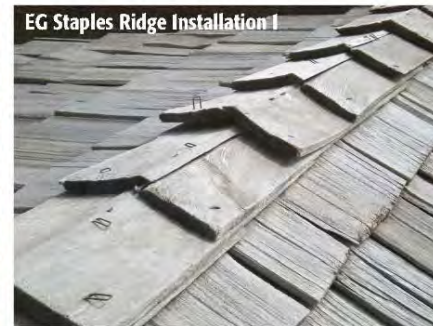
EG Staples Fastener Failure 10-18-11
